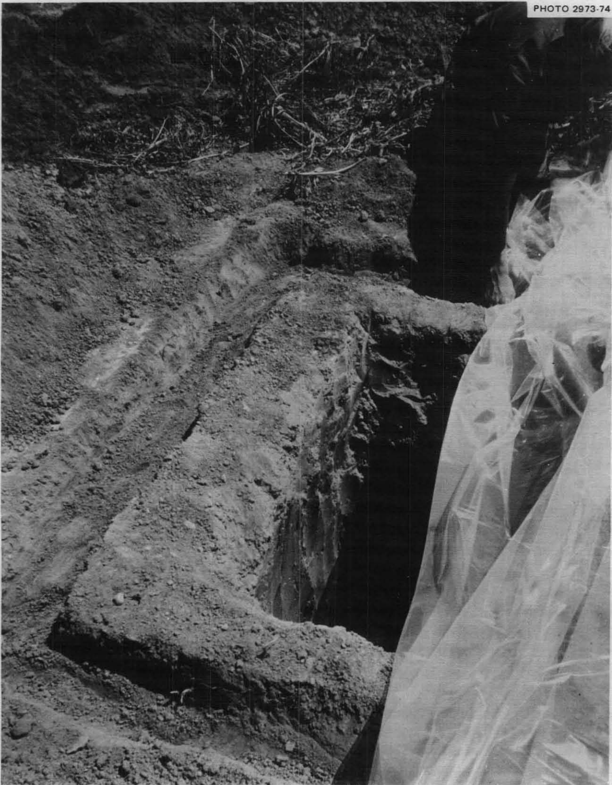
Fig. 4.34. Placing a sheet of 4-mil polyethylene in a 120-gallon water-storage pit. Unlike previous water-storage pits dug and tested by Kearny, this pit was not first lined with cloth or other material to keep sharp roots, etc., from puncturing the waterproofing plastic. All root ends were merely cut off with a knife. The edges of the plastic were folded into the small side trenches, and then held by packed earth. Six days after being filled, no leaks had developed.
